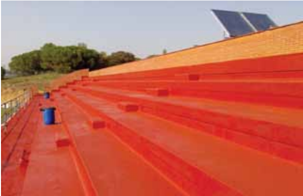
SPAIN Waterproofing of Stadium Tibunes
