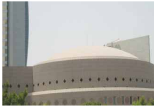
UNITED ARAB EMIRATES-DUBAI Dome Roof
