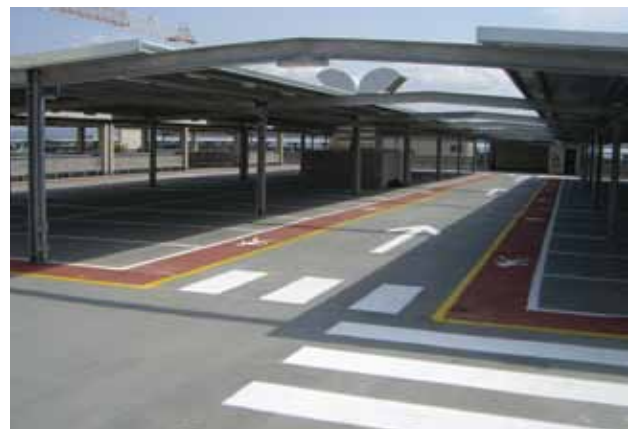
SPAIN Parking Deck, Girona Airport
