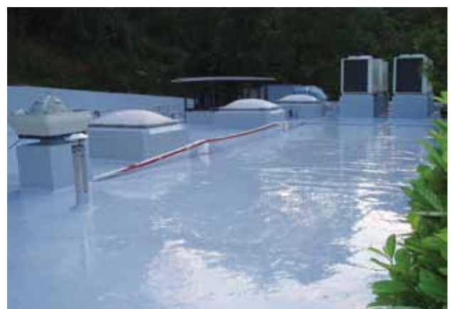
ITALY Flat Roof
