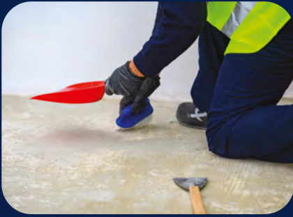
STEP 1 Preparation of the surface
