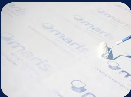
STEP 7 2nd layer of waterproofing membrane
