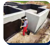
Foundations and retaining walls
