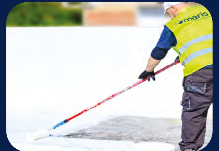
STEP 6 Reinforcement and 1st layer of waterproofing membrane
