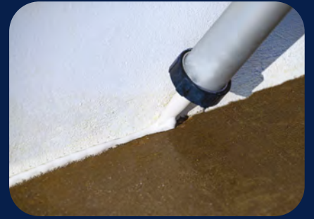
STEP 3 Fixing cracks and joints
